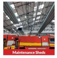
Airius destratification fans work simply and inexpensively alongside all types of HVAC equipment to improve your energy management by balancing temperatures, reducing both heating and cooling costs by between 20% to 50% or more and create gentle air movement throughout the internal space.
